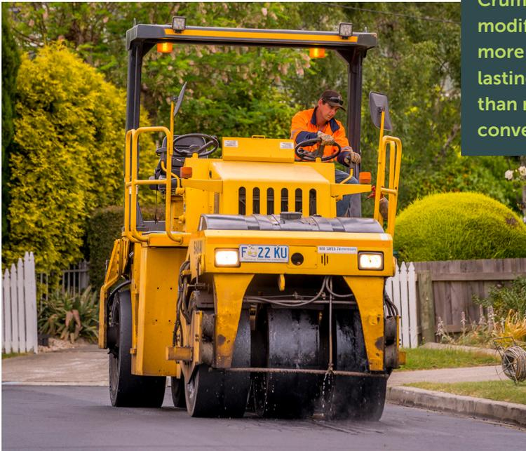
**Crumb rubber modified bitumen is more durable, longer lasting, and quieter than roads paved with conventional asphalt.**
