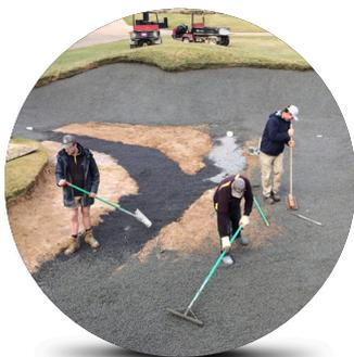
An innovative manufacturer transforms end-of-life tyres into crumb rubber to deliver a hard-wearing, durable, flexible and porous surface. It is the perfect solution for cart paths and bunker linings on golf courses.
