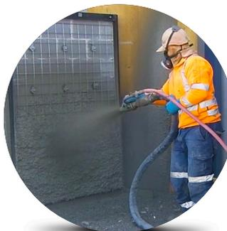
A spray on cementitious mix designed by an innovative manufacturer, made with tyre-derived crumb rubber and composite fibers, is designed to be blast, ballistic and fire-resistant.
