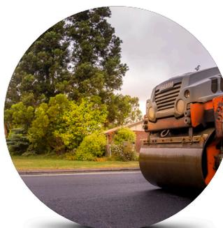
Crumb rubber from end-of-life tyres are being used in high value applications such as road surfacing, ensuring a flexible, porous and long-lasting surface.
