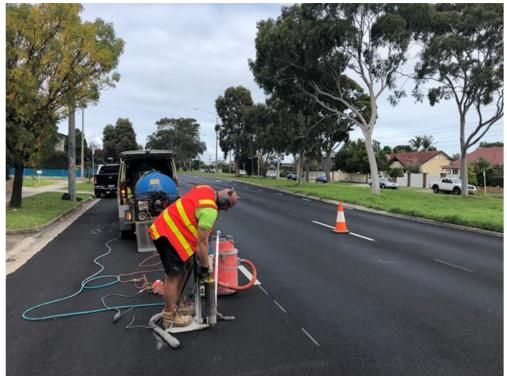
Figure 4.2: Extracting cores from completed trial sections
